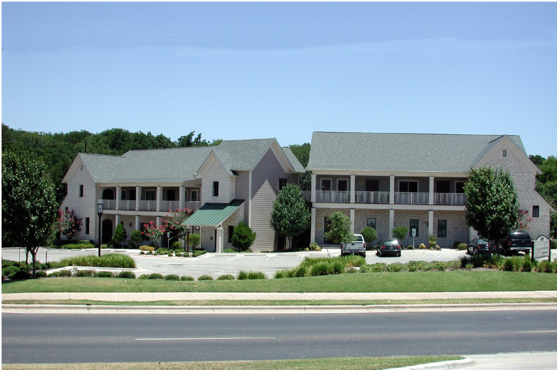
Spicewood Office Condominiums, Spicewood Springs Road, Austin, Texas
